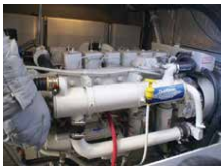
Heat exchanger thermal photo from a Cummins 6BTA5.9 engine. With no discernible areas of temperature variations spotted using thermal imaging the unit was pulled out to find that it was almost 50 % blocked. The gauges never showed any signs of potential overheating and due to the limited hours on the engine there were no plans or indications they needed service.
